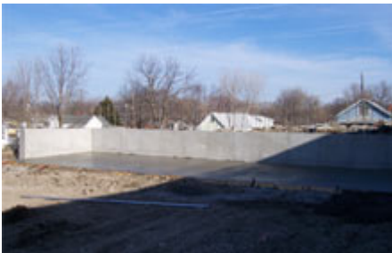
Another view of the start of the new dock area
