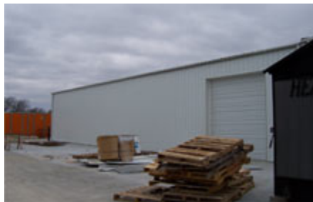
Exterior of the completed new extension on the south side
