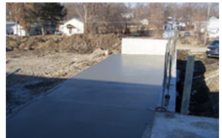
Start of the new dock area
